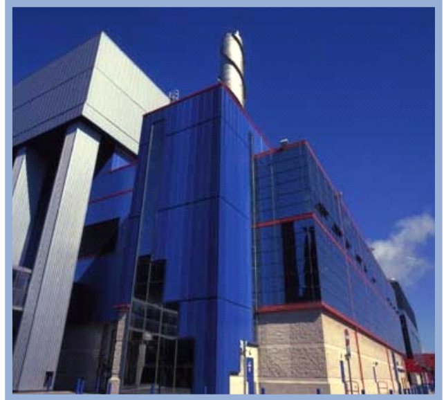
The Waste Packaging and Encapsulation Plant
