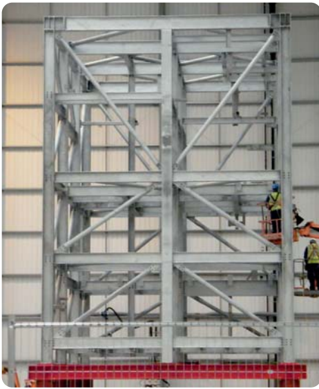
Module Fabrication at Ellesmere Port
