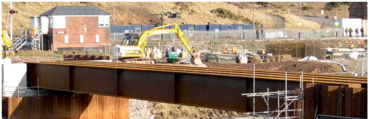
Installation of the bridge beams
