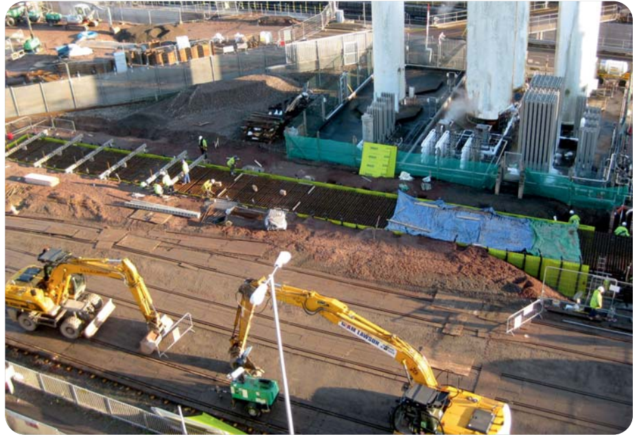
East Gantry Foundation Reinforcement
