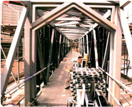
Bridge structure, concrete floor and curtain wall framework components awaiting fitment
