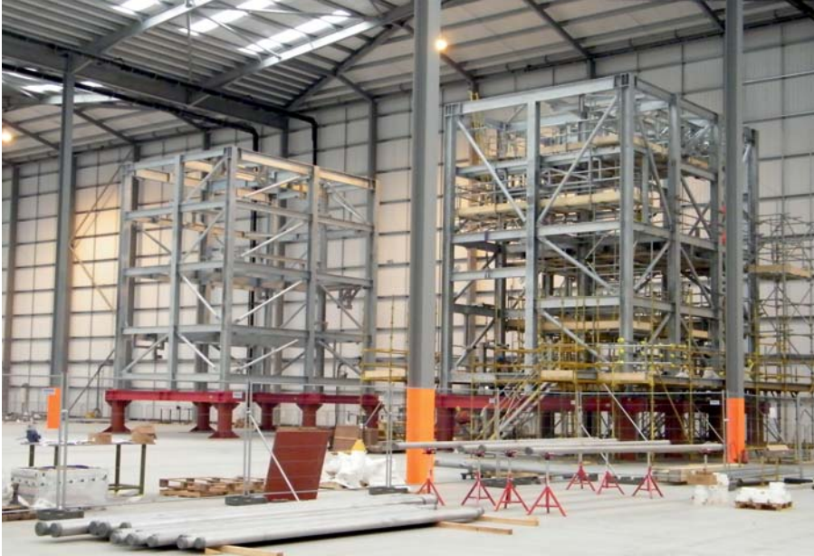
Module fabrication at Pioneer Point, Nr Ellesmere Port
