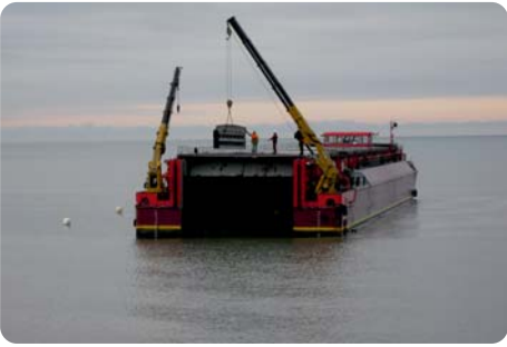
First Panel Removed
