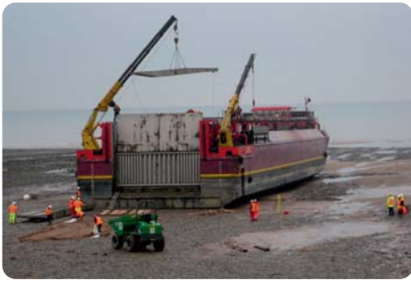
Ramps being lifted down
