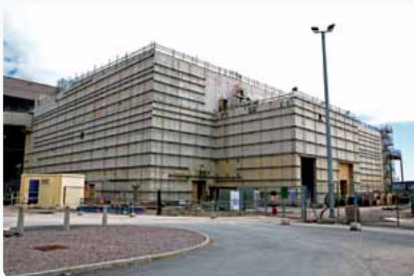
Construction of the new state-of-the-art store for customers' plutonium
