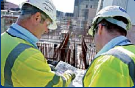
Planning future facilities to support spent fuel management
